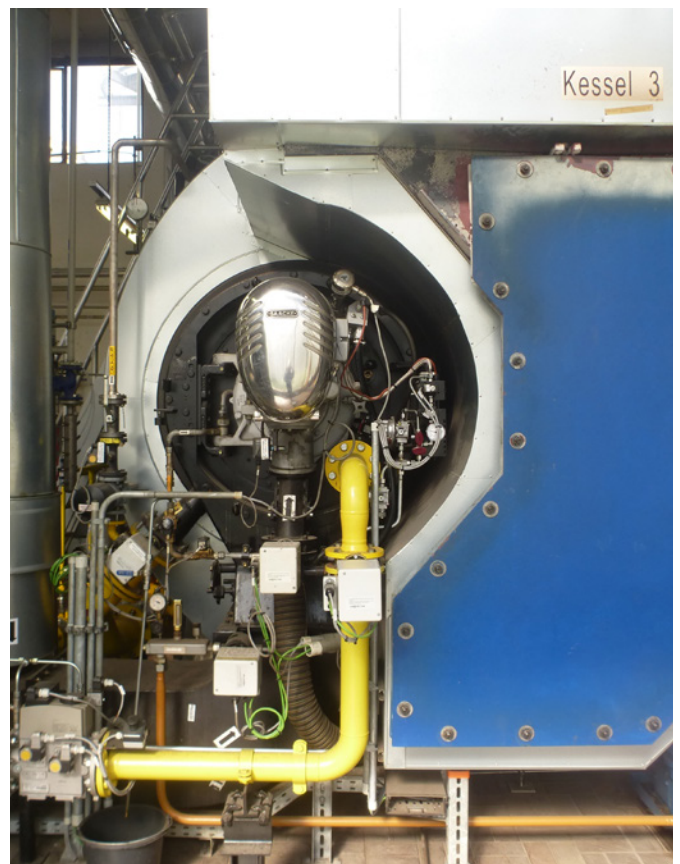
Above: One of the three SAACKE SKVGD hydrogen burners in use at the specialty chemicals company Nouryon in Ibbenbüren
